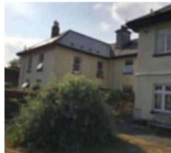
46 - Easton House, Easton
